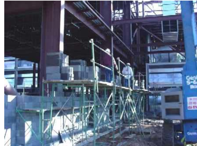
Guardrail Missing
